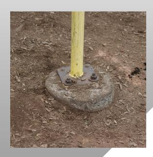
Concrete footings and other anchoring devices should be installed beneath the full depth of safety surfacing.
